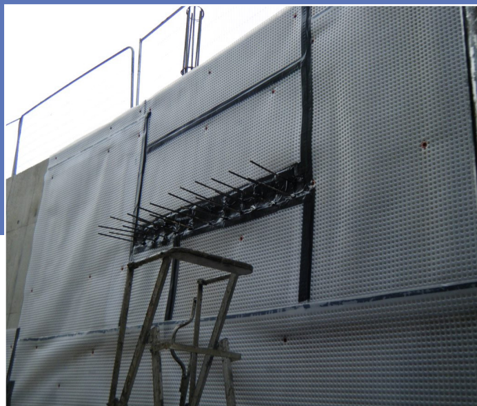
Newton System 500 being used on the basement walls.
