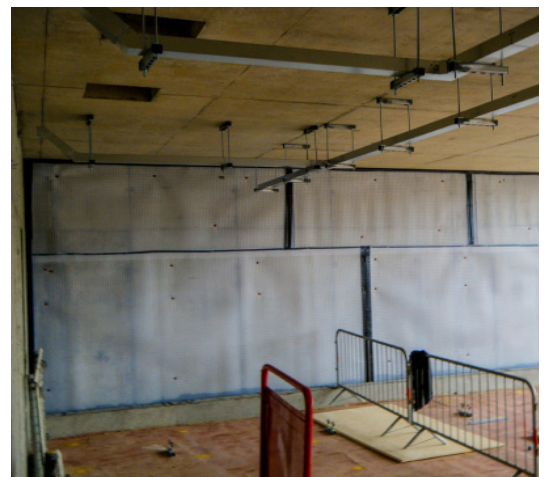
Newton 508 membrane applied to the walls.
