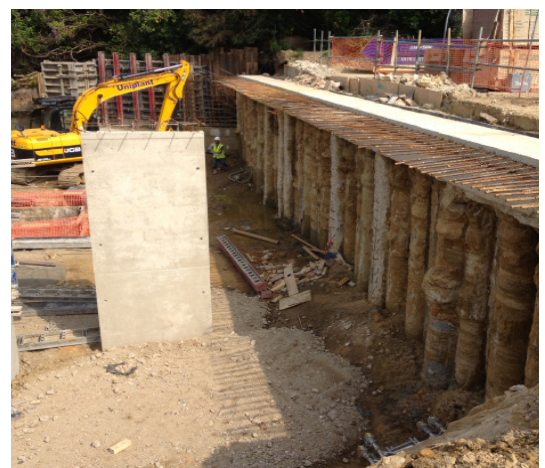
Early stages of basement construction.
