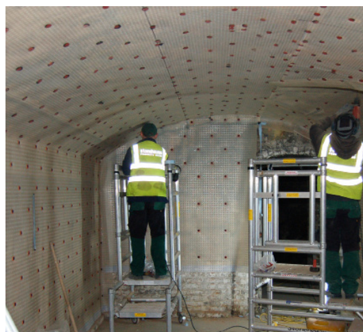
Newton 508 Mesh being expertly installed.
