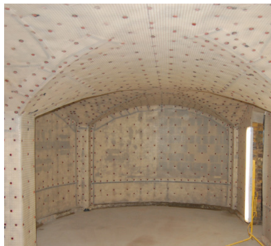
Completed installation of Newton 508.
