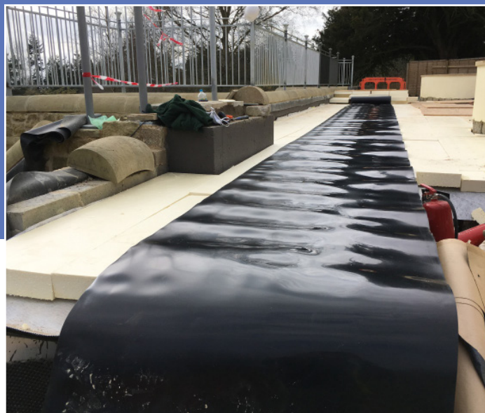
Installation of Newton 409 RootBarrier .
