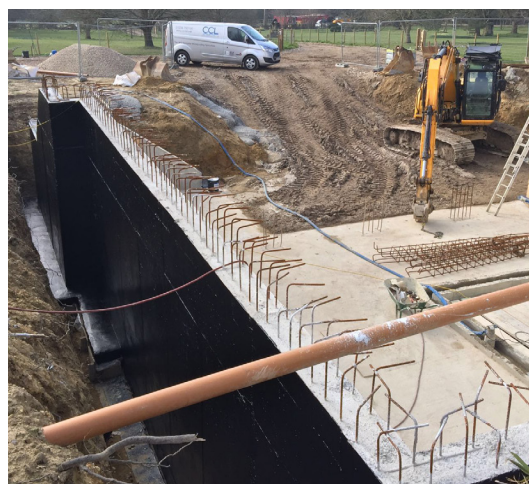
Continuous external waterproofing protection.
