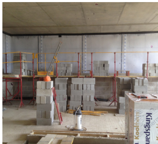
Newton System 500 installed to the wall and floors.
