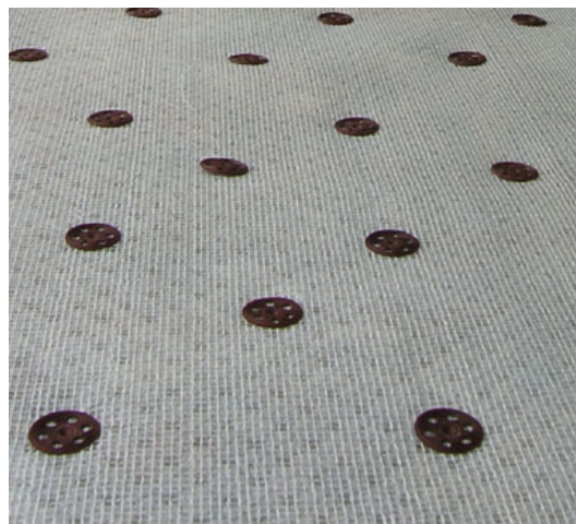
The mesh is heat-welded into the membrane.
