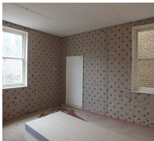
Newton 803 Newtonite membrane was installed.
