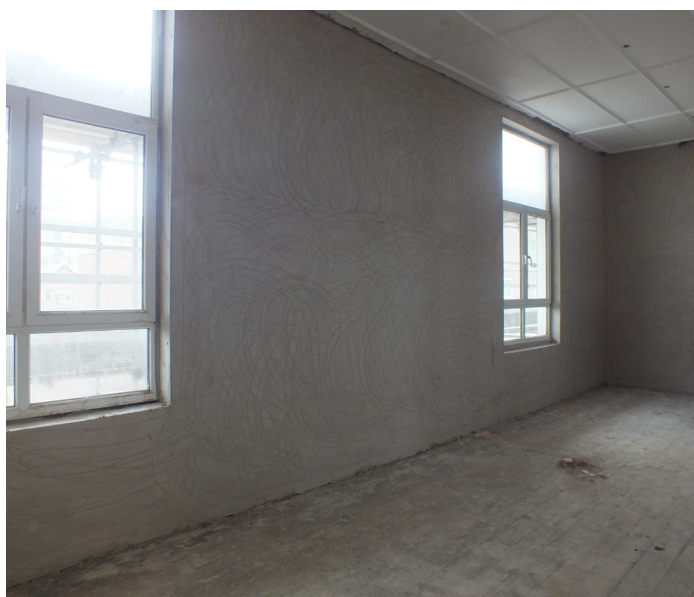
Plaster was applied directly to the membrane.
