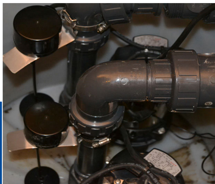
The Dual Pumping System comprised of two NP750 Pumps.
