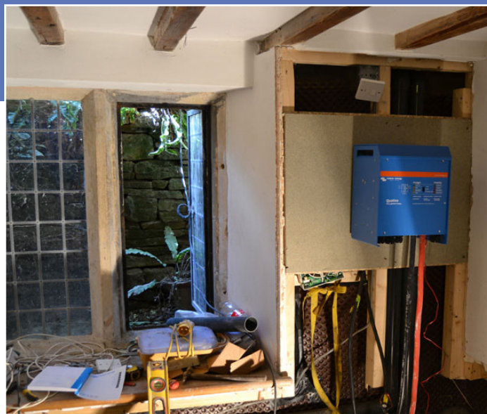
The Victron Inverter was installed temporarily at the start of the project.
