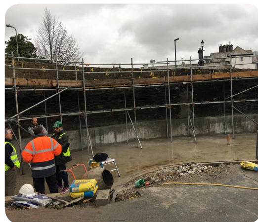
2. The new building was an unusual shape, with Phase 1 taking the form of a large curved structural wall
