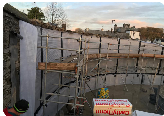
5. Despite the size of the project, Premier delivered the waterproofing installation quickly and efficiently
