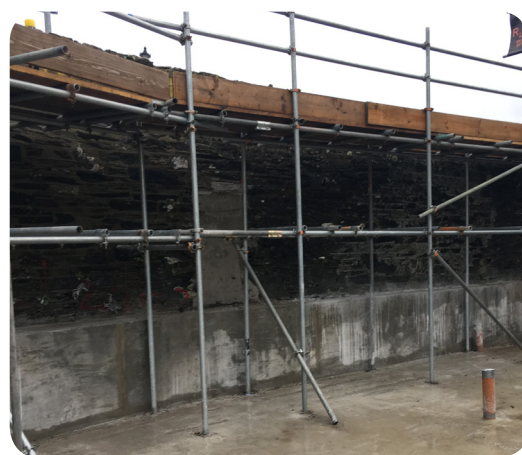
1. The large, uneven new structure was ideal for the flexible, resilient 109-LM liquid membrane
