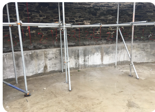
3. When planning their cavity drain install, Premier also had to account for the wall's large concrete kicker
