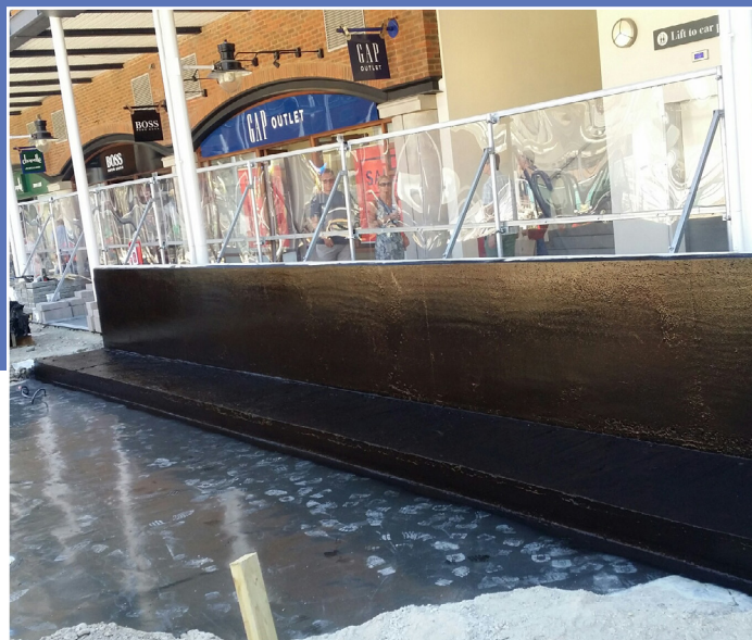
The rubber waterproofing was hand and spray applied to the substrate.
