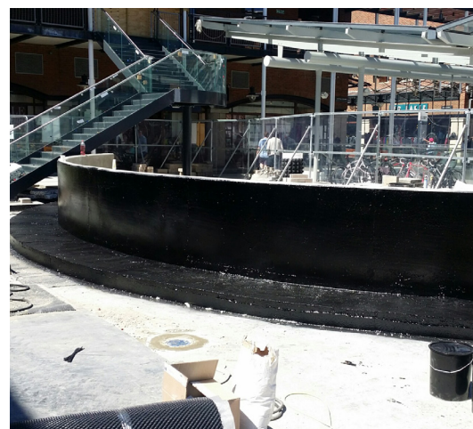
Application was to retaining walls and adjacent deck areas.
