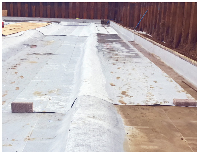
When placed below a new raft, the poured concrete engages into the locking fleece
