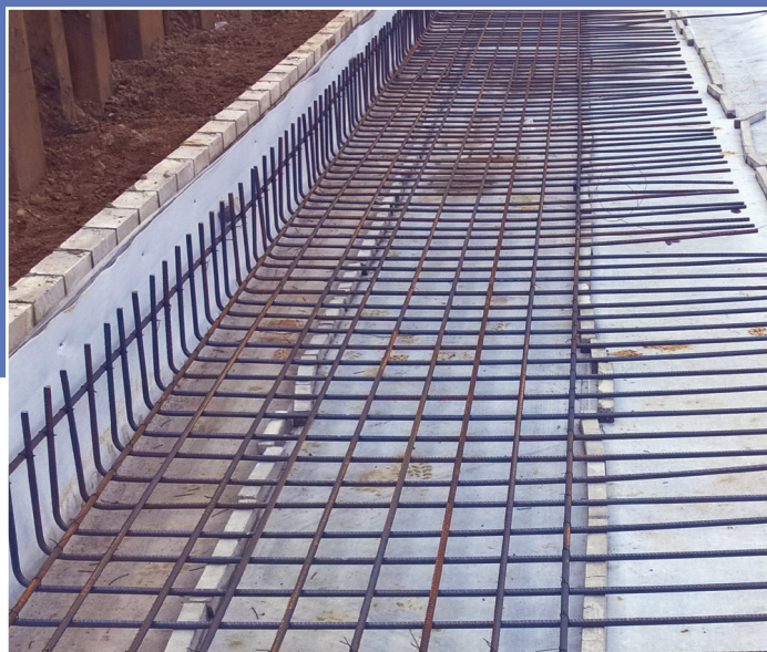
For good practice, concrete spacers are placed on top of the 70mm lap to reinforced this joint
