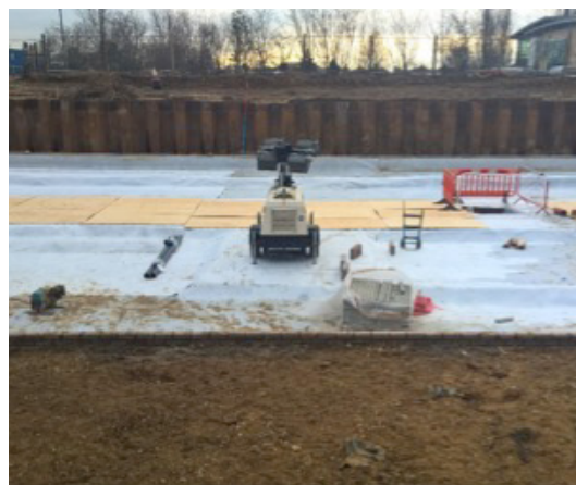
403 HydroBond is a self-healing waterproof membrane
