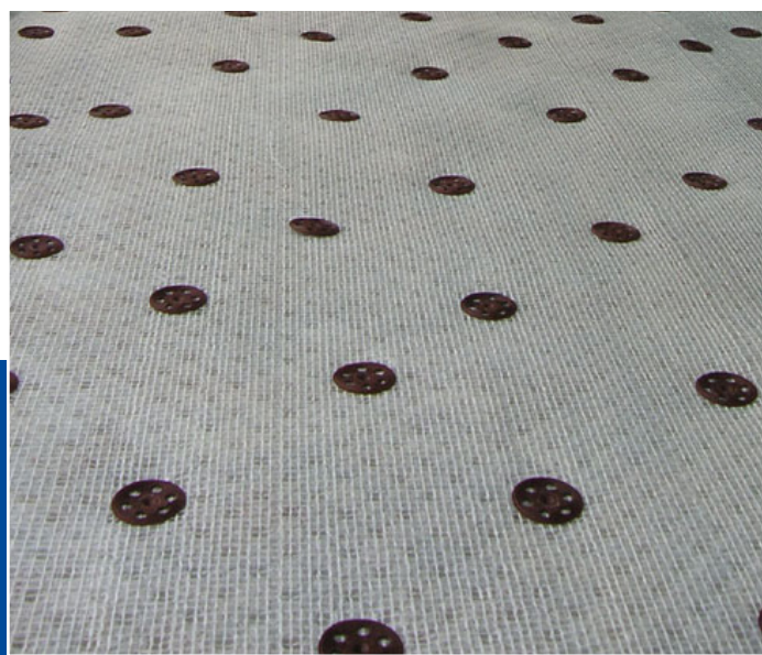
Newton 805 Newlath was the ideal solution to the damp problem.
