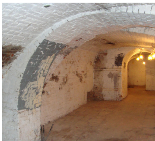
Convoluted damp walls prior to treatment.
