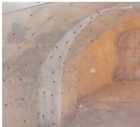
Application of Newton 508 mesh to vaulted areas.
