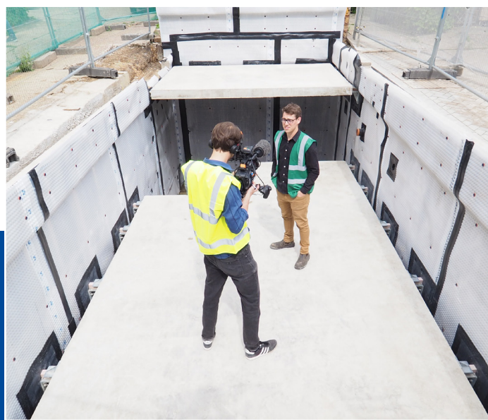
The final System 500 waterproofing installation.
