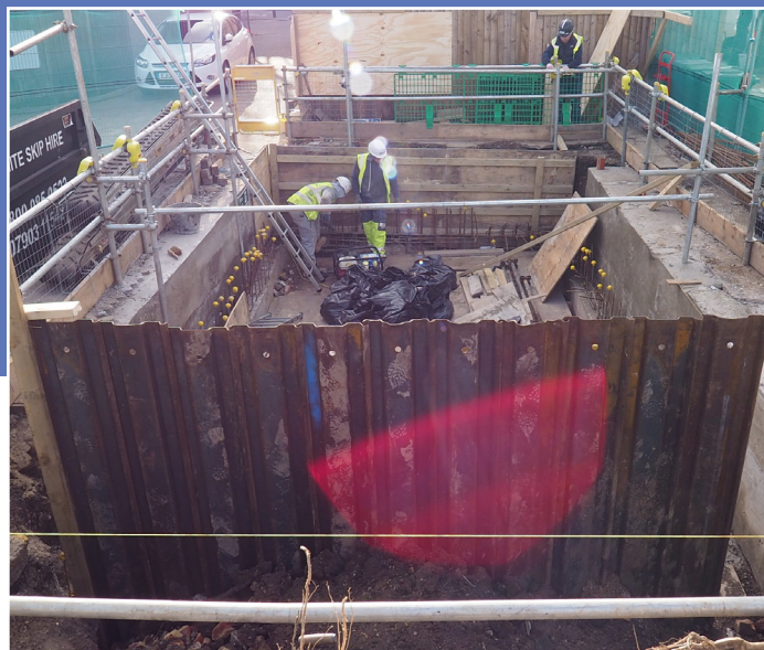
The new excavation was properly supported with sheet piles.
