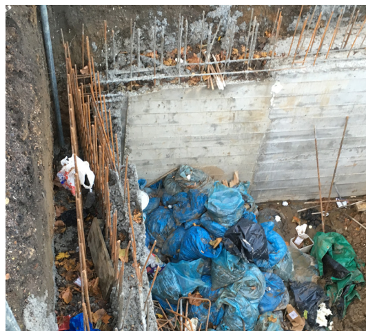
Compacted concrete had burst the shutters.
