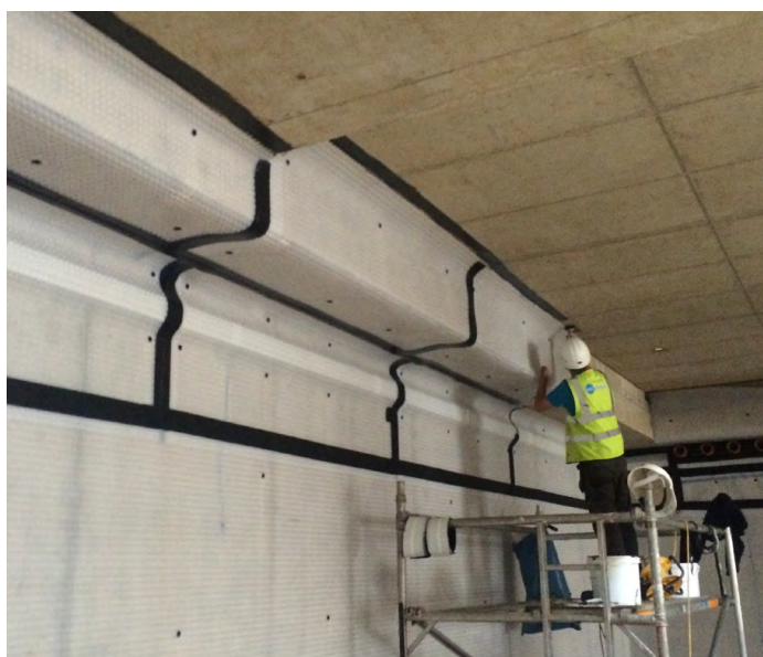
The duct was then fitted around the basement to deliver air pressure
