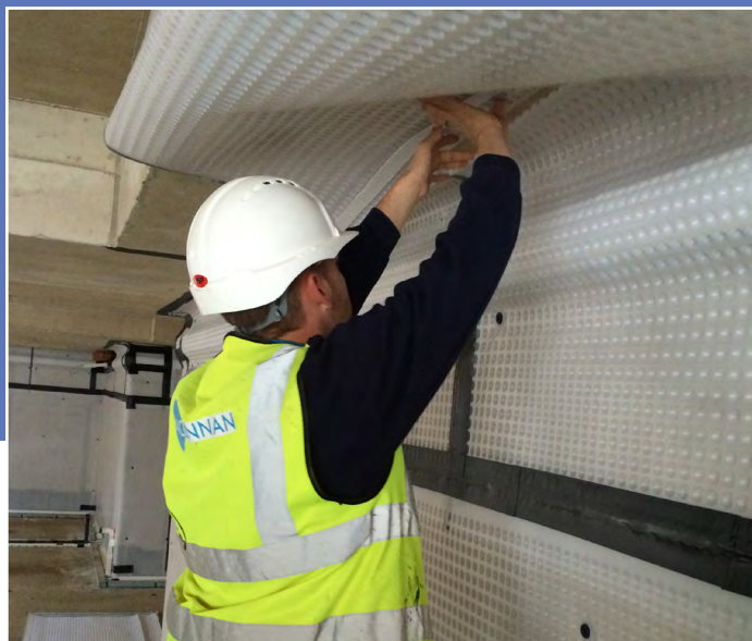
MacLennan's trained installers fitted the Newton cavity drain membrane
