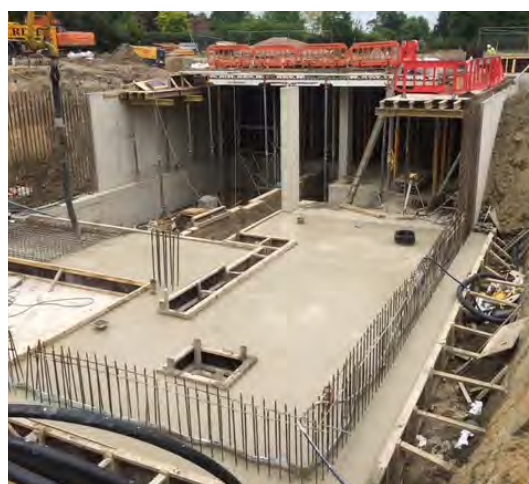
The 4-metre deep new concrete basement
