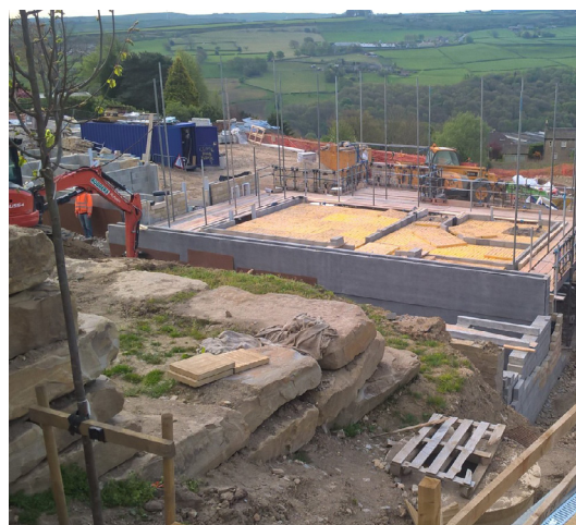
The blockwork ready to be waterproofed.
