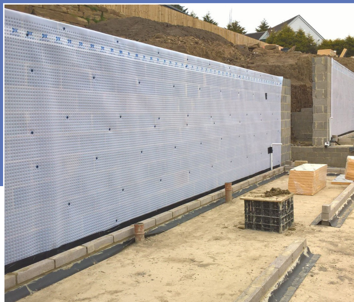
Type A external and Type C internal waterproofing was required.
