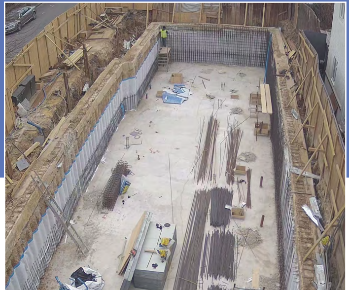
With the slab poured, 403 HydroBond continued up the walls.
