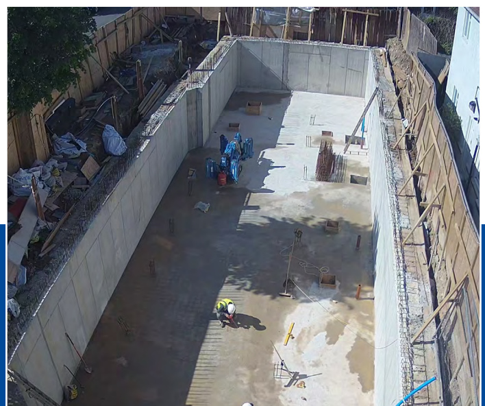
A pristine concrete basement with two types of waterproofing complete.
