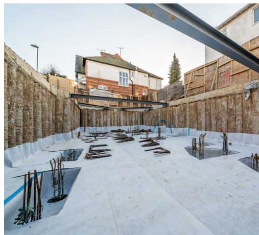
403 HydroBond installed beneath the concrete slab.
