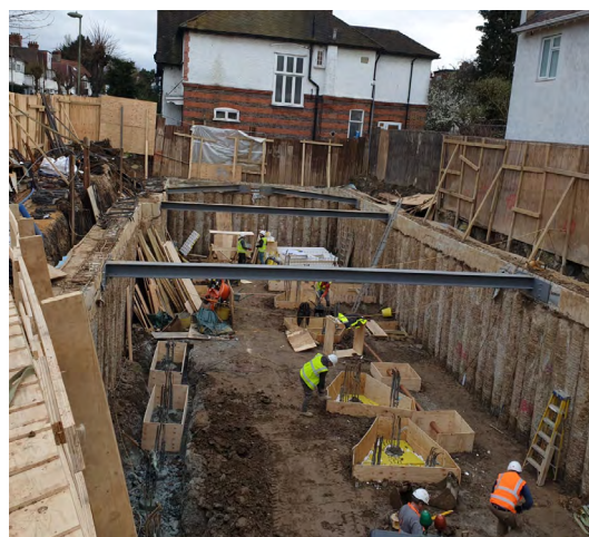
Arti Construction installed 267 secant piles on the site.
