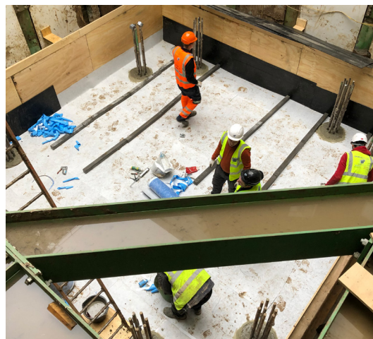
Installing HydroBond prior to a concrete slab install
